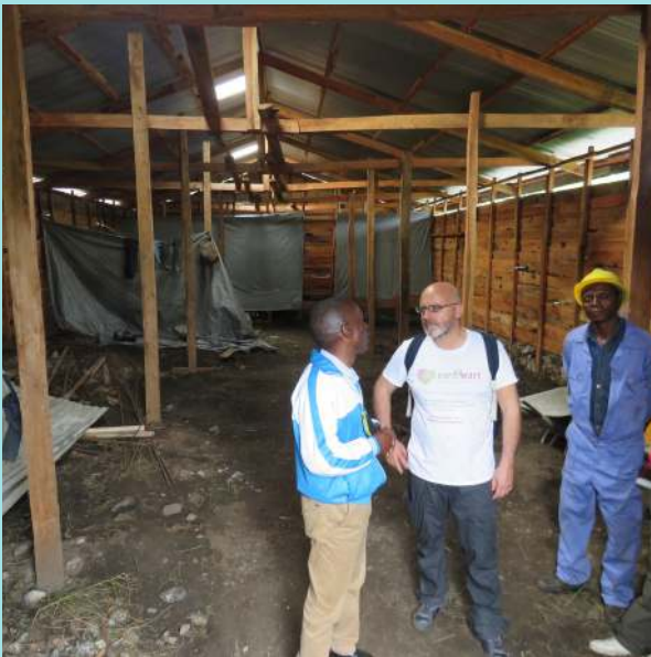
Alberto talking with Kizungu and the engineer inside the poultry house
